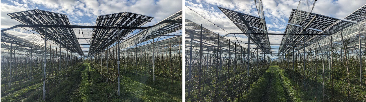
Figure 1: Fixed angle (left) and tiltable (right) mounting system equipped with semi-transparent photovoltaic panels.
